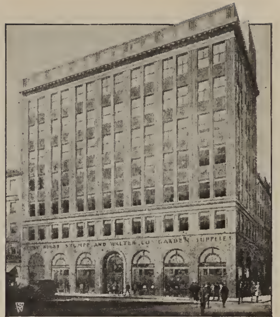
Ideal storage facilities are provided in our New York headquarters. Here, and at our branches, we are equipped to serve you personally.
